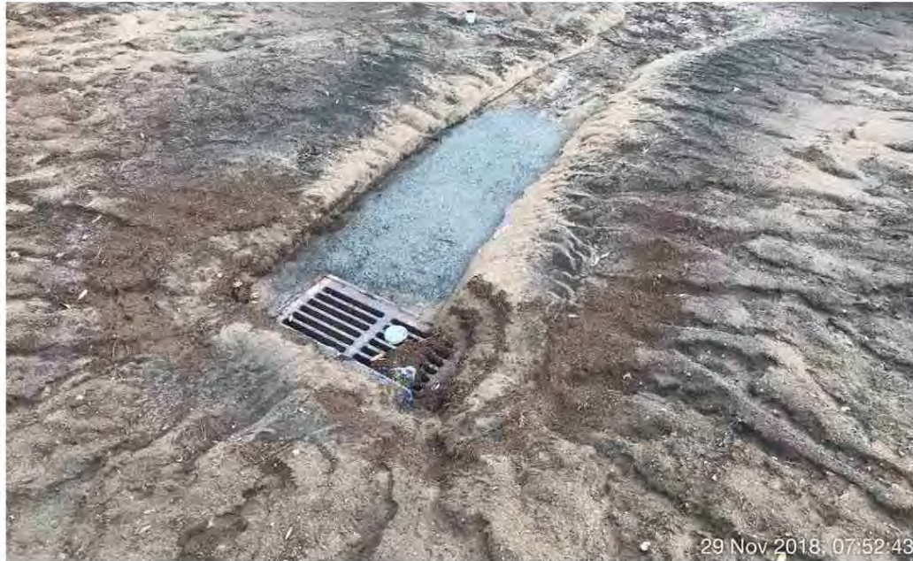
Photo 5. Pond outlet structure, 11/29/18
