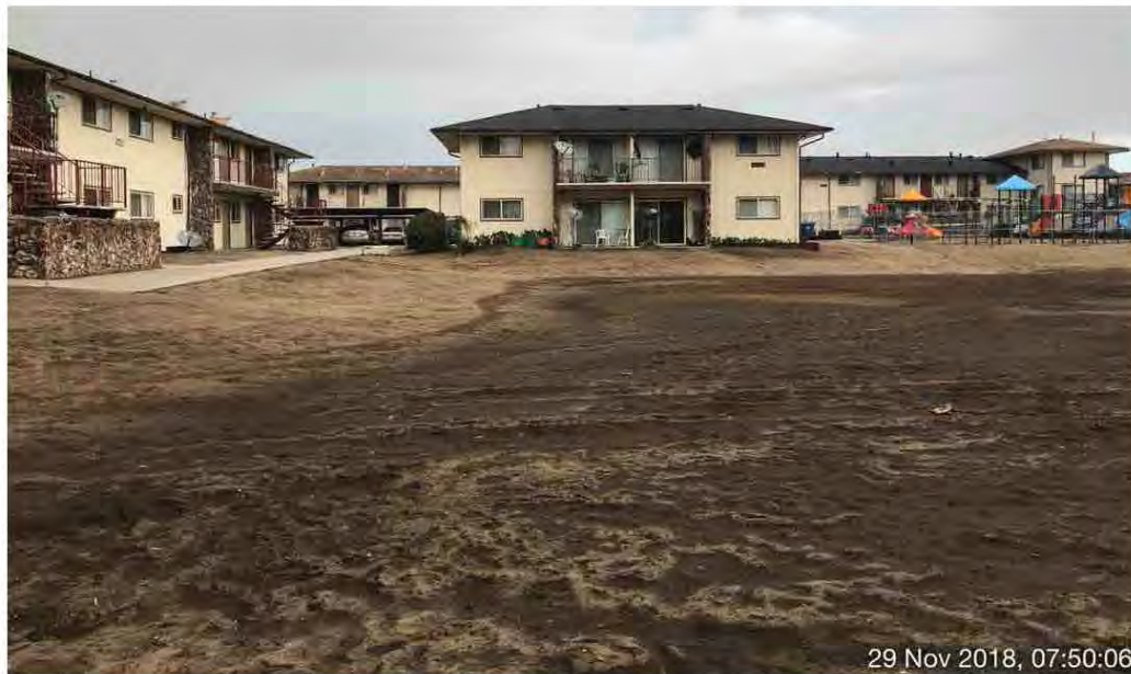
Photo 7. Debris deposition across pond bottom, 11/29/18
