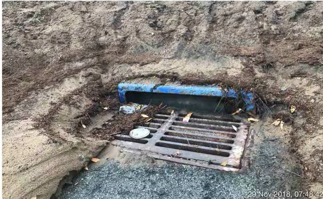
Photo 6. High water mark at pond outlet structure, 11/29/18
