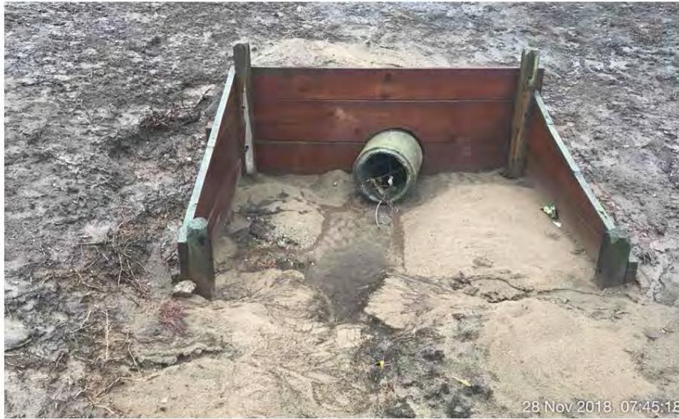
Photo 3. Pond inlet pipe, 10/28/18
